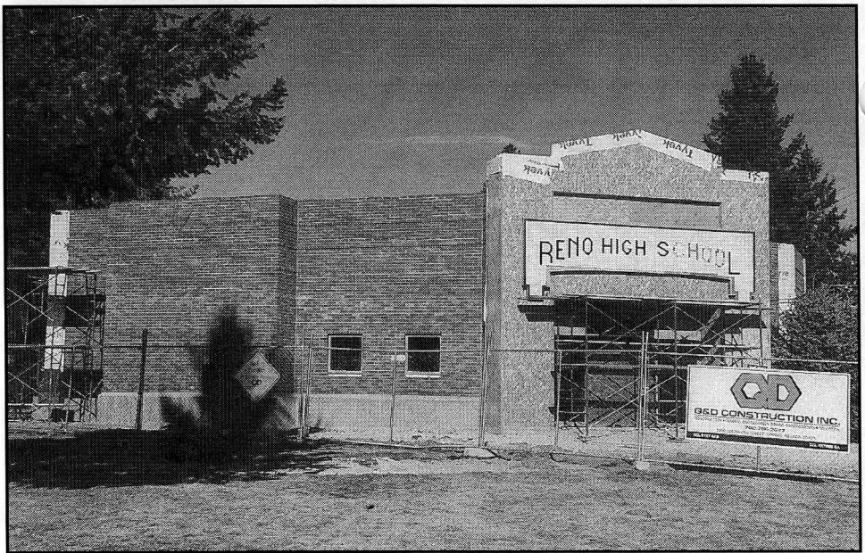
Exterior of building, prior to finishing touches.
